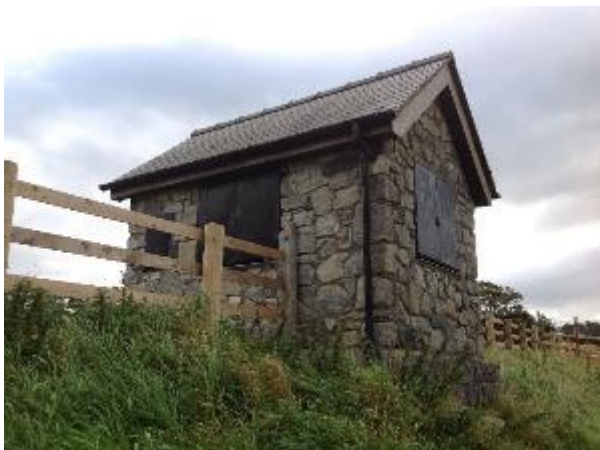
PICTURE 5. BUILDING AT TN5.
