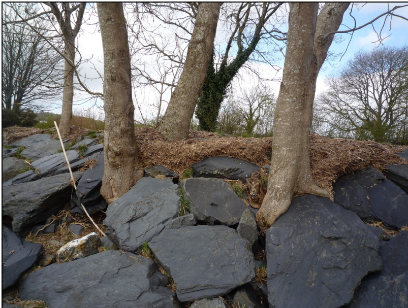
P5 – Embedded rocks/boulders at base of stems on group 4. These cause potential fracture points when trees are loaded or during inclement weather
