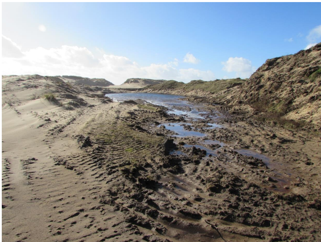
Photograph 25. Wet slack in the Phase 2 area, deepened as part of the Phase 3 works, looking west
