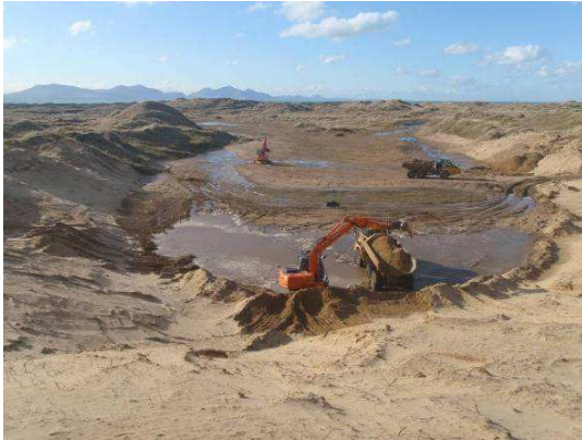
Photo 1: Excavation in progress in Slack 2 (E1 in this report) 11 th March 2013.
