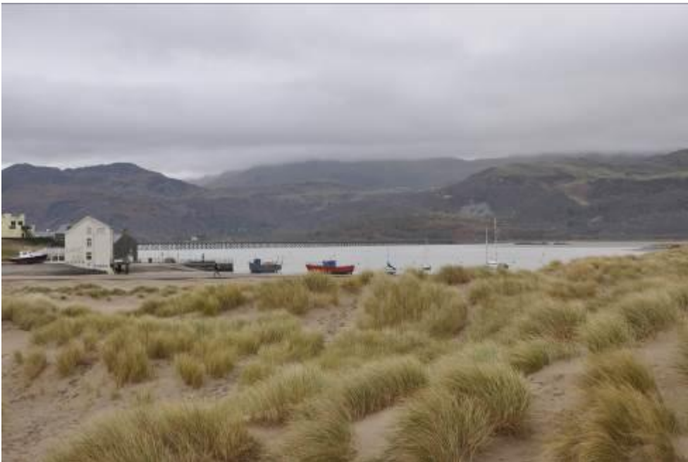
Barmouth railway viaduct and wooden trestle bridge
